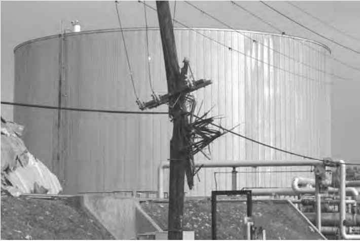
Figure 4.1.15 Utility Pole - Hurricane Rita (Photo Courtesy of FEMA)
