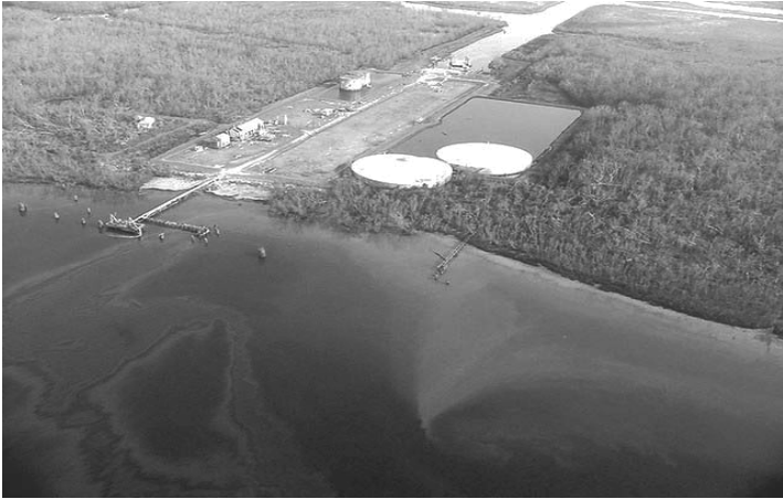
Figure 4.1.8 Oil Storage Tanks – Hurricane Katrina (Photo Courtesy of NOAA)
