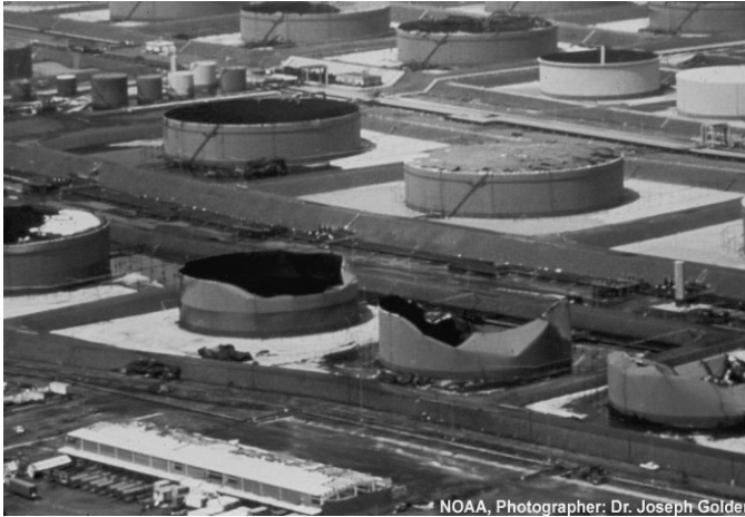
NOAA, Photographer: Dr. Joseph Golden Figure 4.1.2 Petroleum Storage Tanks – Hurricane Hugo (Photo Courtesy of NOAA)
