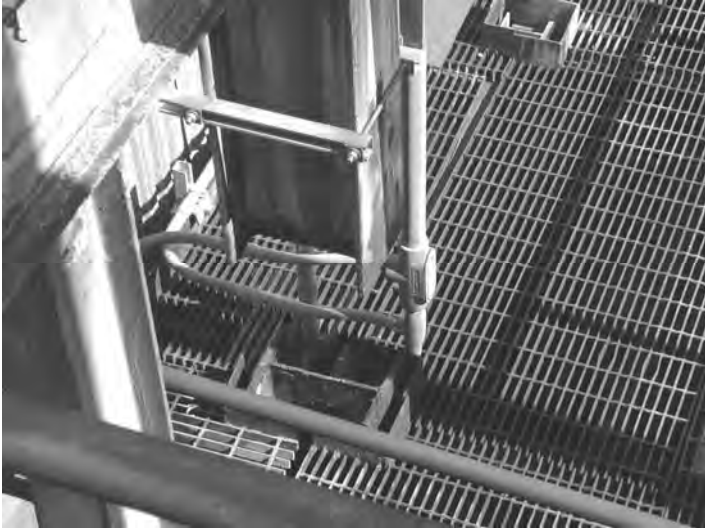
Figure 4.6.2 Photo of a Field Modification to an Existing Steel Column
