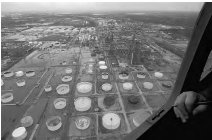
Figure 4.6.1. Aerial Photo of Typical Petrochemical Facility (Courtesy of FEMA)
